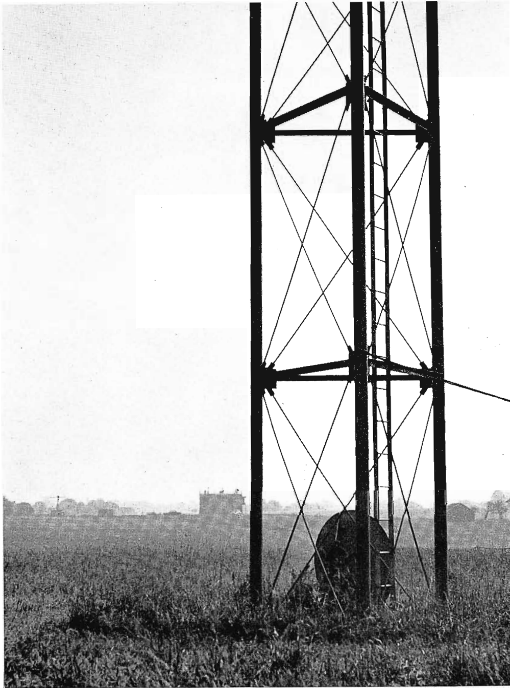
An existing tower (also see photo at right) at the Camden Test Site provided various heights for mounting "dish" receiving antenna. Rotating pedestal and test house can be seen in the background at extreme lower left.
