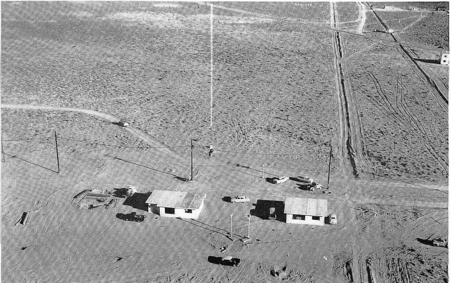
Aerial view of test site showing radio building at right, and 150-foot guyed antenna.
