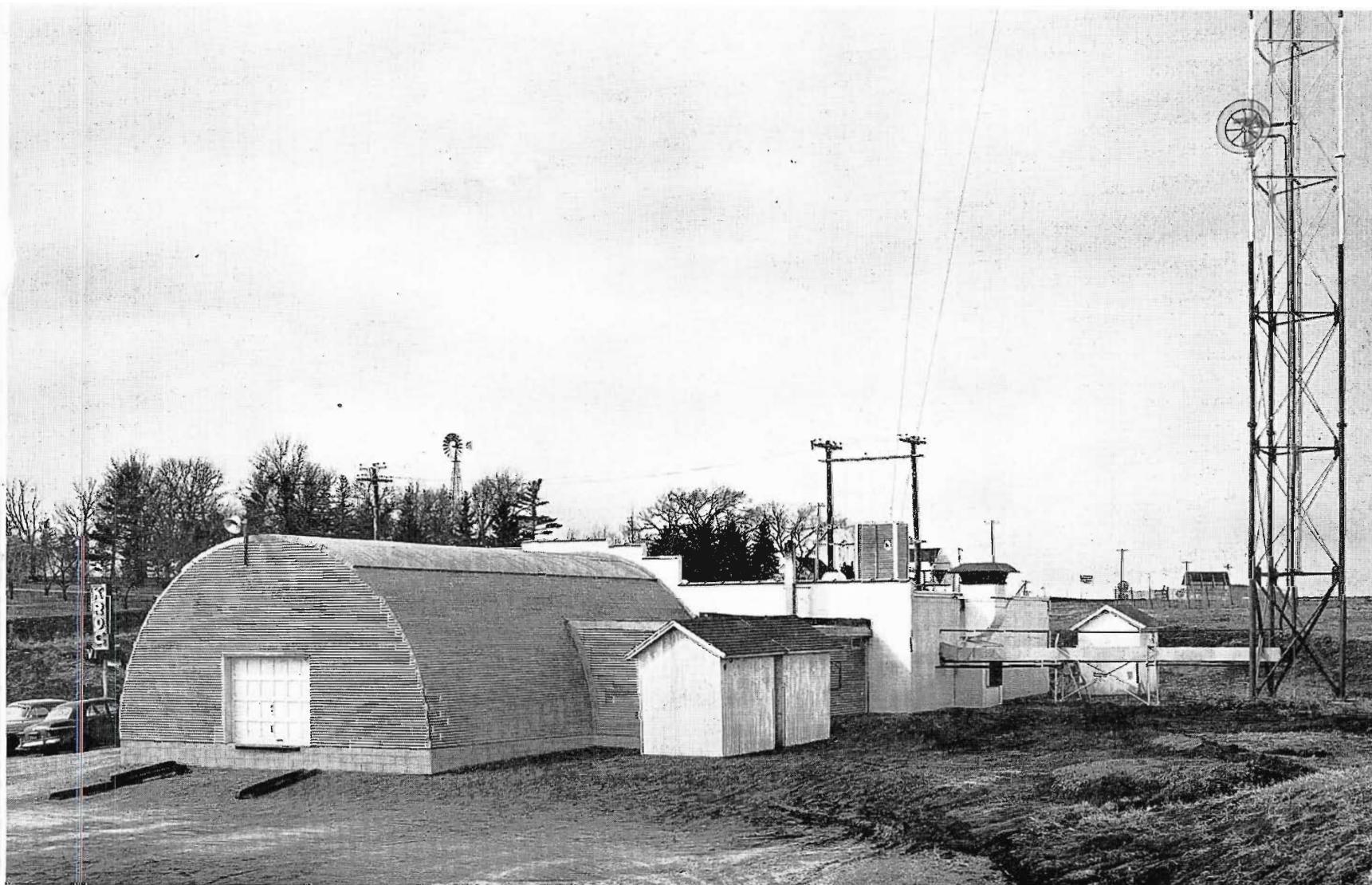
FIG. 12. Looking southwest—Quonset studio with modification. Small sheds are used for additional prop storage. Parts of portable ramp can be seen lying in front of studio door. Dish antenna 50 feet up on tower is AT&T microwave equipment to bring NBC network shows.
