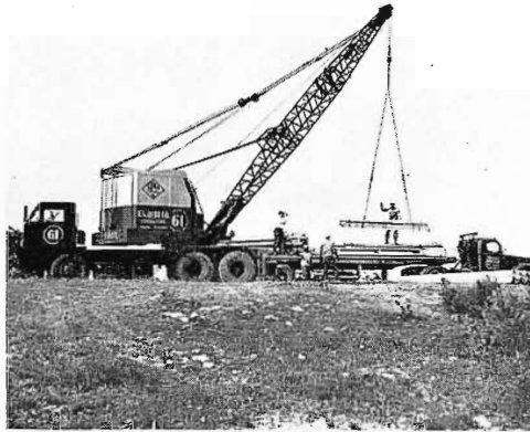
Tower diagonal-bracing members are unloaded from trucks at the stockpile area.
