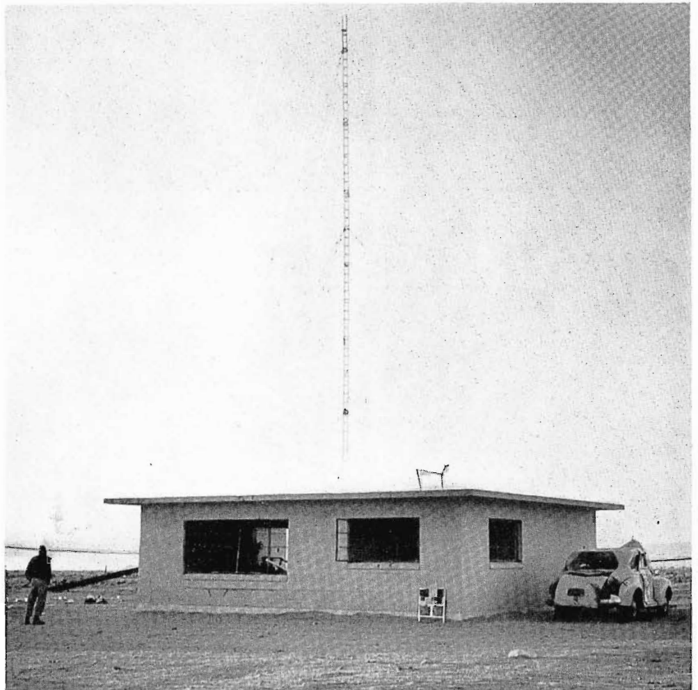
Concrete block house after the blast—TV antenna is down, windows are blown out, car is badly damaged, mahogany doors became toothpicks, but the house stood up—so did the transmitter.
