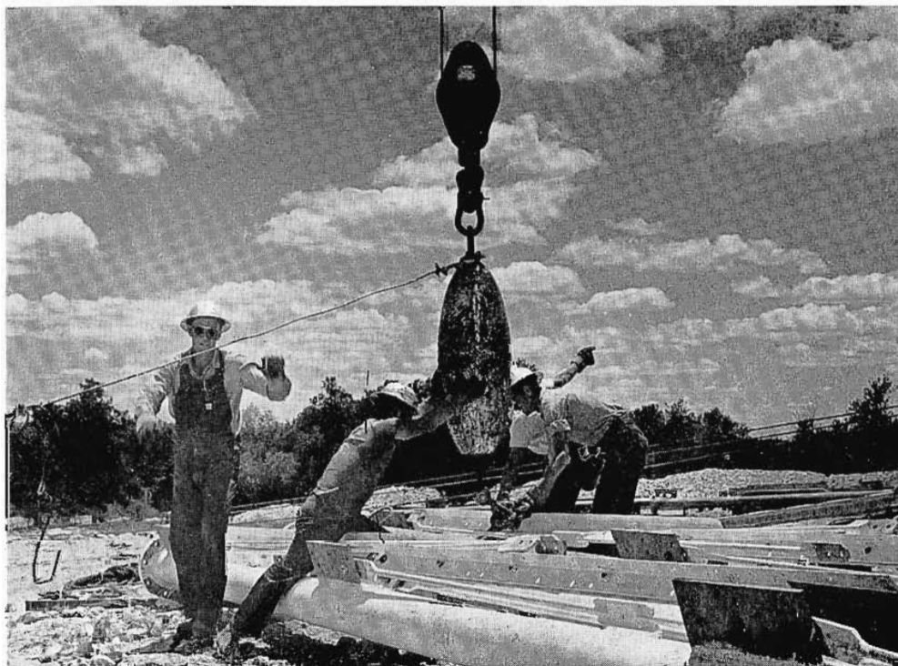
One of many typical guy anchorage piers with steel plates in place.
