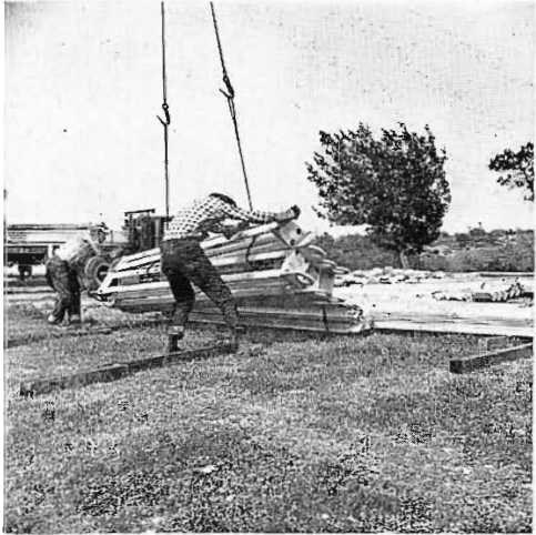
Orderly layout of tower components proceeds with skillful handling.
