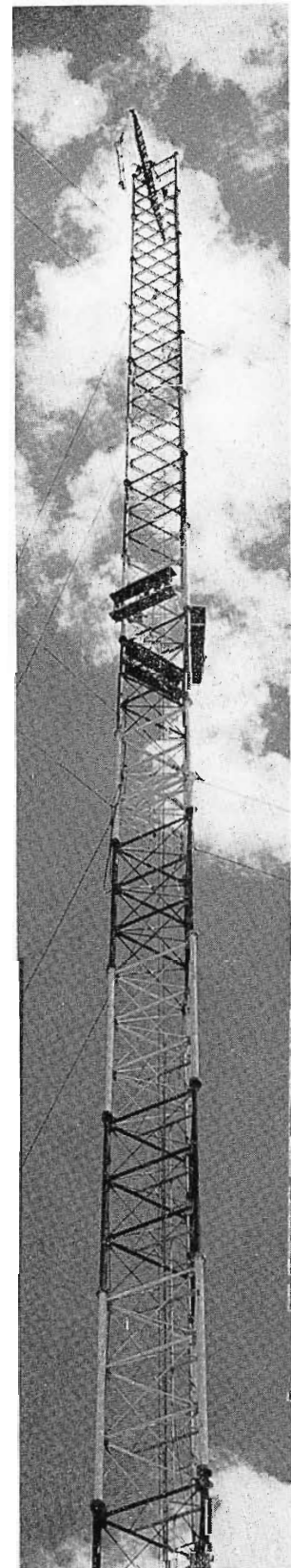
Nearing half-way mark the pattern of the tower structure repeats itself every 30 feet.
