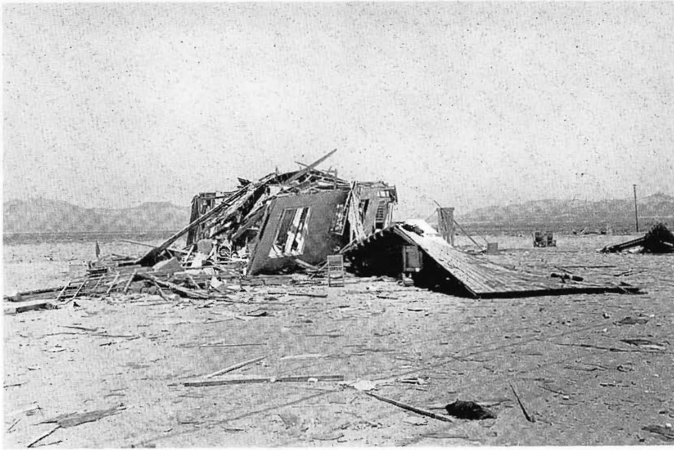
Frame house after the blast—the building was completely demolished.
